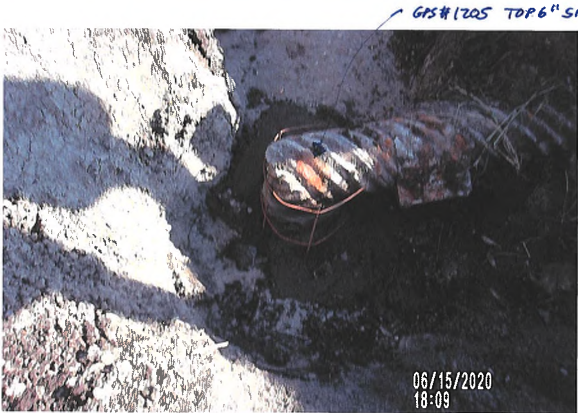
PICTURE # 3762 IS LOOKING SOUTH SHOWING 1.0' X 2.0' 6" X 6" WIRE MESH AROUND 6" TO 8" CMP SPIRAL CONNECTION BEFORE CONCRETE POURED.
