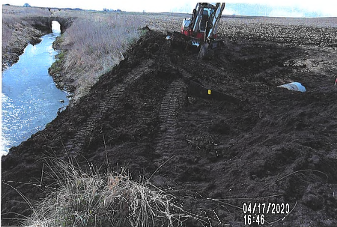
PICTURE #3394 IS LOOKING NW SHOWING CREW BACKFILLING DRAINAGE DITCH BANK AROUND 36" CMP & HDPE ANTISEEP COLLAR
