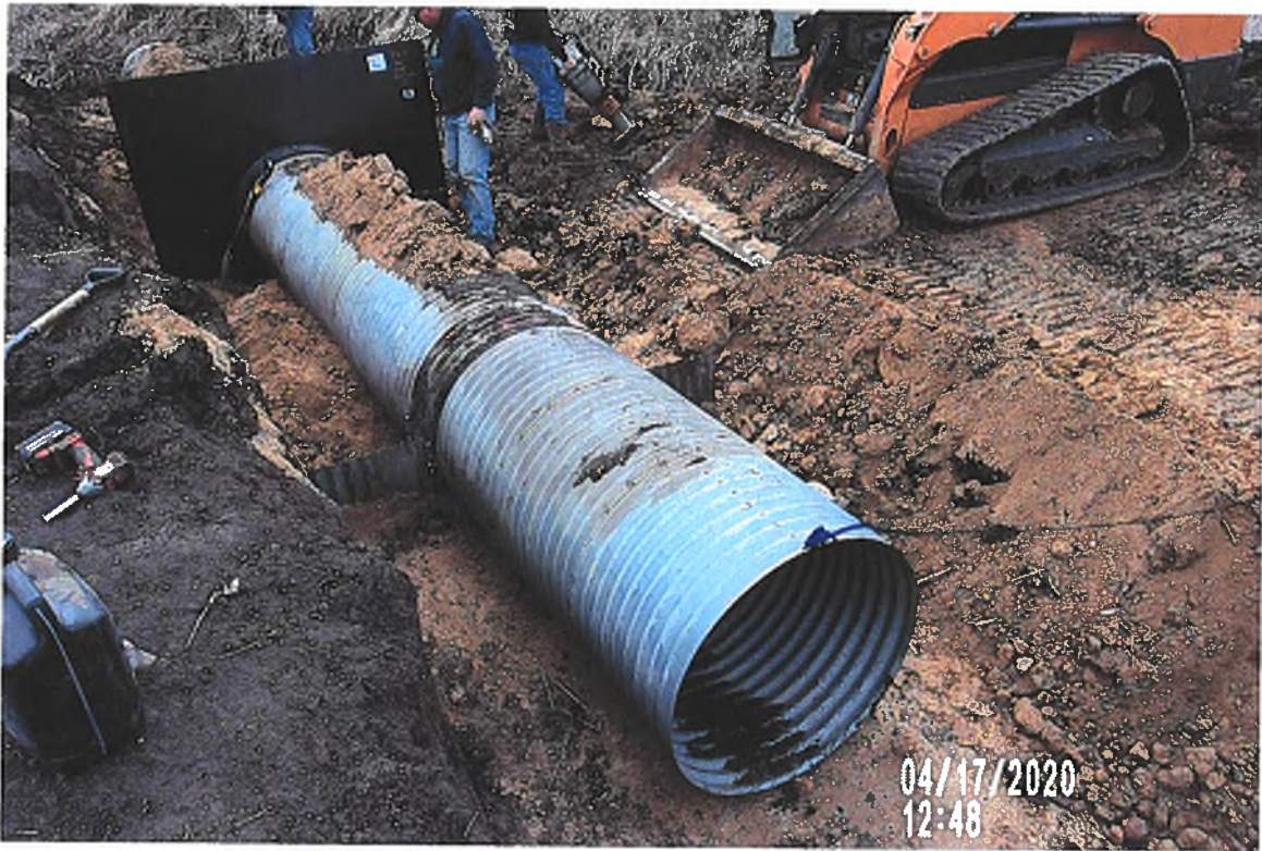
PICTURE#3383 IS LOOKING SW SHOWING HDPE ANTI SEEP COLLAR IN PLACE 18.4' ± SE OF NORTH END OF 36" CMP SURFACE DRAIN.
