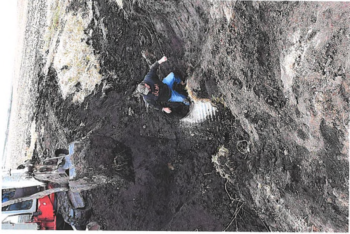
PICTURE # 17 IS LOOKING NW SHOWING CREW REMOVING EXISTING METAL ANTI SEEP COLLAR
