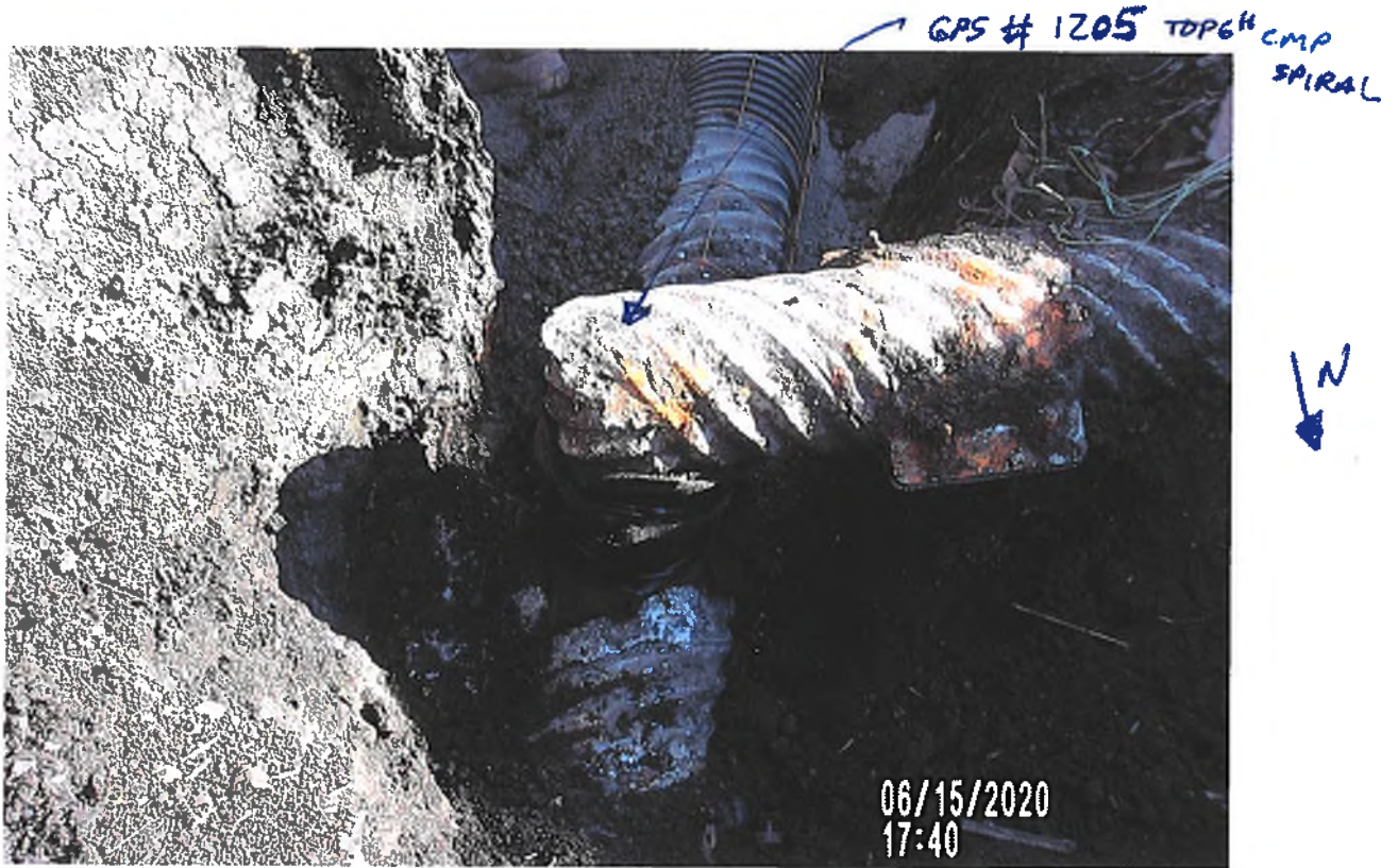
PICTURE # 3759 IS LOOKING SW SHOWING 6" 90° CMP SPIRAL TIE IN INTO 8" CMP SPIRAL WRAPPED WITH FABRIC & TILE TAPED BEFORE CONCRETE COLLAR POURED,
